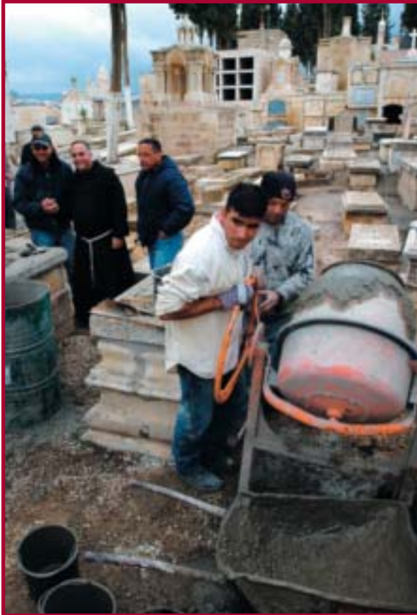
Fr. Amjad Sabarra, OFM, looks on as workers repair parish cemetery.
